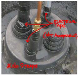
Always check your pipe portals after the installation of each pipe. Make sure that they are using the correct strap and they are installed tight
